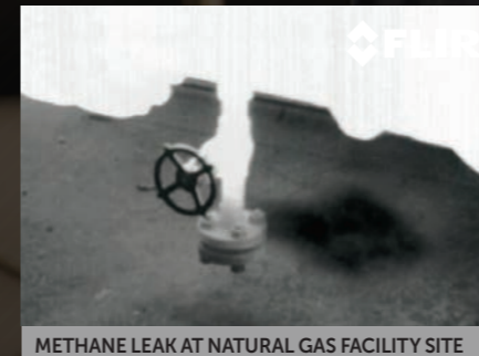
METHANE LEAK AT NATURAL GAS FACILITY SITE
