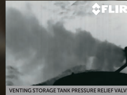
VENTING STORAGE TANK PRESSURE RELIEF VALVE
