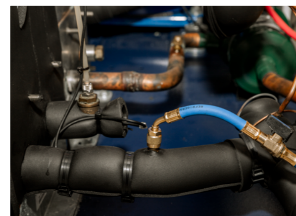
Connection hoses with ball valves for quick closing and opening of refrigerant flow.
